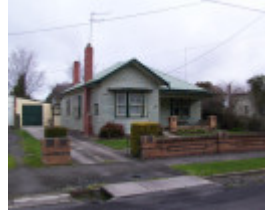
14 Steinfeld Street South
