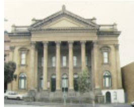
1 masonic hall bendigo front view
