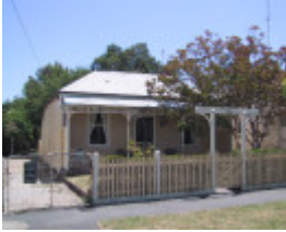
320 Raglan Street South
