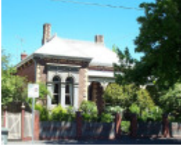
239 Lydiard Street North
