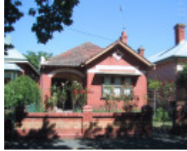
114 Raglan Street South
