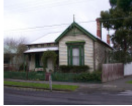
12 Steinfeld Street South
