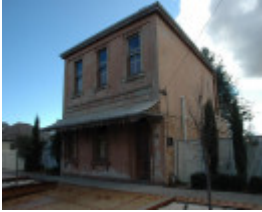
Former Post & Telegraph Office, Moorabool Shire Heritage Study Stage 1, 2010
