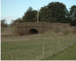
Navigators Railway Bridge, Moorabool Shire Heritage Study Stage 1, 2010
