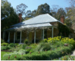
Mine Manager's House, Moorabool Shire Heritage Study Stage 1, 2010
