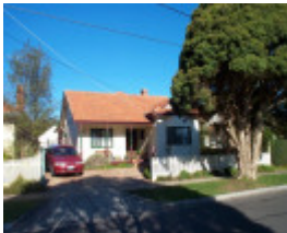
House at 6 Elliston St
