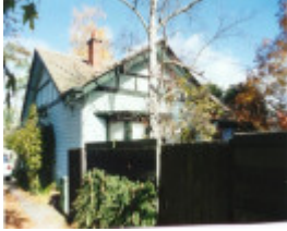
House at 298 Mount Dandenong Rd
