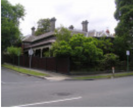
Review of B Graded Buildings in Kew, Camberwell & Hawthorn
