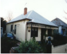
House at 12 Wilana St
