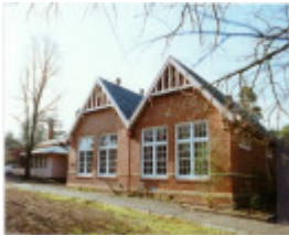
Croydon Community School
