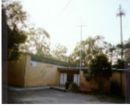
Bedford Road Scout Hall
