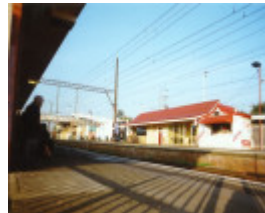
Ringwood Railway Station
