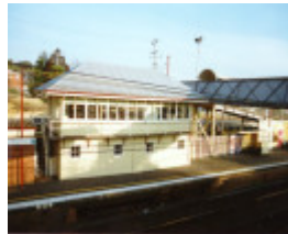
Ringwood Railway Station
