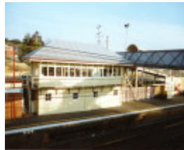
Ringwood Railway Station
