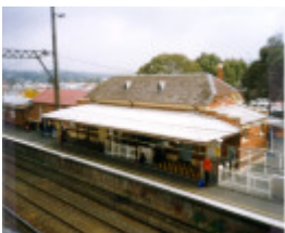
Maroondah Hwy, Ringwood Railway Station.jpg
