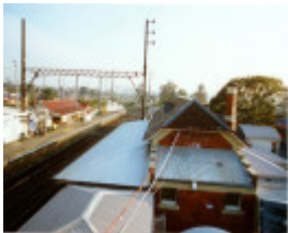
Ringwood Railway Station
