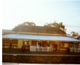
Ringwood Railway Station
