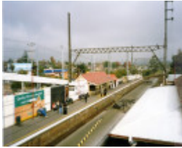
Ringwood Railway Station
