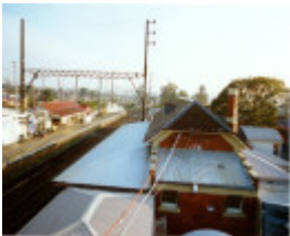
Ringwood Railway Station
