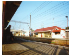
Ringwood Railway Station
