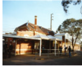
Ringwood Railway Station
