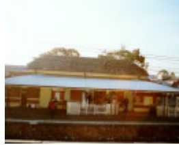
Ringwood Railway Station
