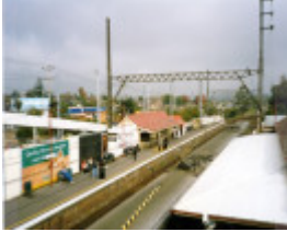
Ringwood Railway Station
