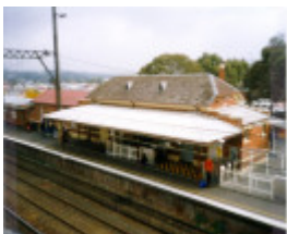
Maroondah Hwy, Ringwood Railway Station.jpg
