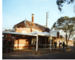
Ringwood Railway Station
