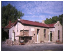
former bendigo gas works bendigo residence office
