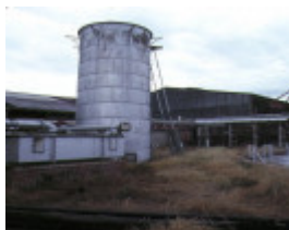
former bendigo gas works bendigo silo mar1989
