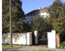
Review of B Graded Buildings in Kew, Camberwell & Hawthorn
