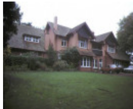
1 edrington berwick front view of house apr1985
