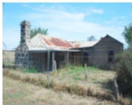
JOHN KELLY'S FORMER HOUSE SOHE 2008
