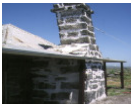
john kelly's former house whiteside street beveridge restored chimney nov1993
