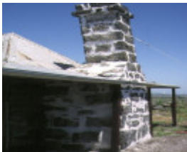
john kelly's former house whiteside street beveridge restored chimney nov1993
