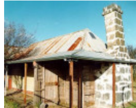
john kelly's former house whiteside street beveridge chimney 2
