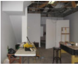
Leitrim hotel interior ground floor looking north
