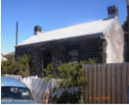
25 Albert Street, Hobsons Bay Heritage Study 2006
