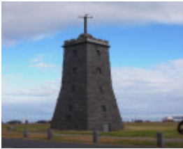
Point Gellibrand Lighthouse (former), Bay Heritage Study 2006
