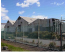
Shell Oil Complex, Hobsons Bay Heritage Study 2006
