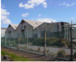
Shell Oil Complex, Hobsons Bay Heritage Study 2006
