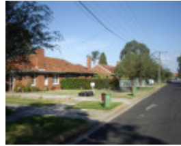
Munition Workers Housing Heritage Area, Braybrook
