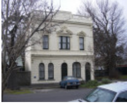
George Hotel (former), Hobsons Bay Heritage Study 2006
