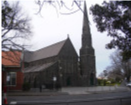
St Mary's Roman Catholic Church Complex, Hobsons Bay Heritage Study 2006
