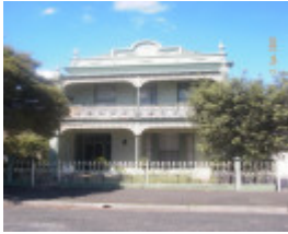
160 Cecil Street, Hobsons Bay Heritage Study 2006
