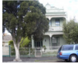
160 Cecil Street, Hobsons Bay Heritage Study 2006
