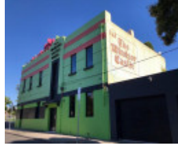
89 Albert Street, Windsor
