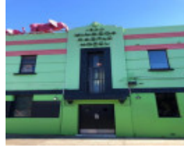
89 Albert Street, Windsor
