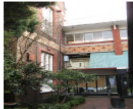
Alfred Hospital Aug 26 2011 KJ east side.jpg
