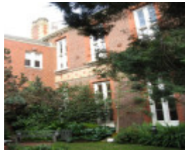
Alfred Hospital Aug 26 2011 KJ east side.jpg
