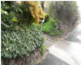
811 Sydney Rd - retaining wall
