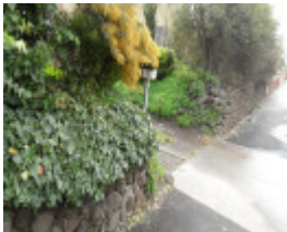
811 Sydney Rd - retaining wall
