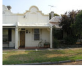
10-16 Davies Street, Hobsons Bay 2006/2007 precinct images No 10
