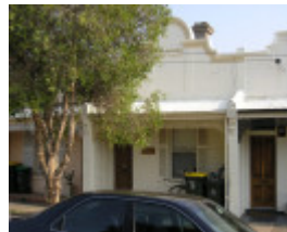
10-16 Davies Street, Hobsons Bay 2006/2007 precinct images No 14
