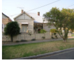
10-16 Davies Street, Hobsons Bay 2006/2007 precinct images No 11
