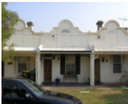
10-16 Davies Street, Hobsons Bay 2006/2007 precinct images No 12
