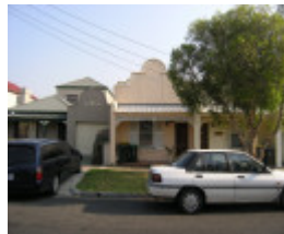
10-16 Davies Street, Hobsons Bay 2006/2007 precinct images No 16
