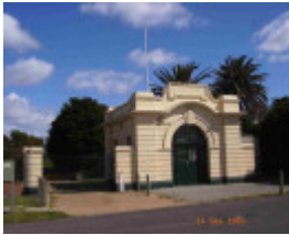
Newport A & B Power Station Gatehouse (former) and Canary Island Palms, Hobsons Bay Heritage Study 2006
