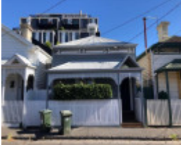
72 Aberdeen Road, Prahran
