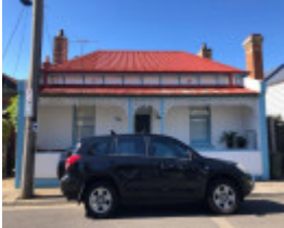
73 Aberdeen Road, Prahran
