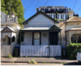
78 Aberdeen Road, Prahran
