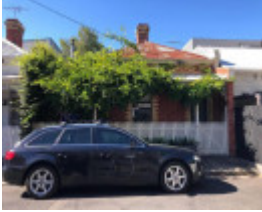
79 Aberdeen Road, Prahran
