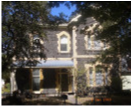
Wesleyan Methodist Manse and Kindergar (former), Hobsons Bay Heritage Study 2006
