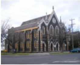
Wesleyan Methodist Church (former), Hobsons Bay Heritage Study 2006
