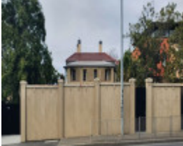
480 Punt Road South Yarra
