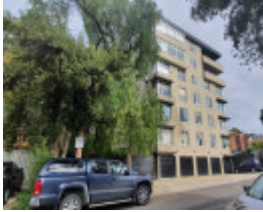
504 Punt Road South Yarra
