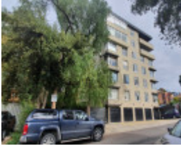
504 Punt Road South Yarra
