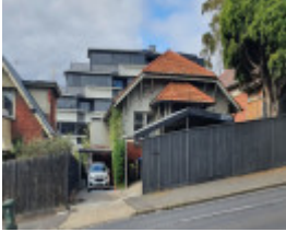
508 Punt Road South Yarra
