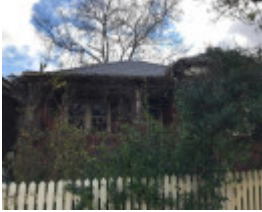
1 Auburn Grove, Armadale
