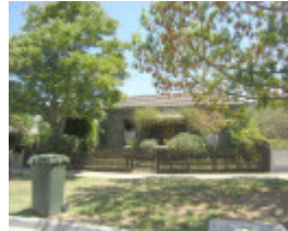
House at 15 Elizabeth Street NEWPORT, Hobsons Bay Heritage Study 2006
