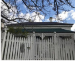
7 Auburn Grove, Armadale
