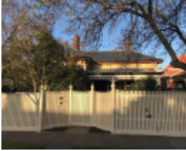
8 Auburn Grove, Armadale
