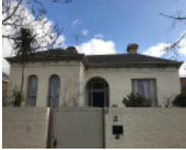
11 Auburn Grove, Armadale
