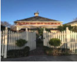
12 Auburn Grove, Armadale
