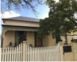
13 Auburn Grove, Armadale
