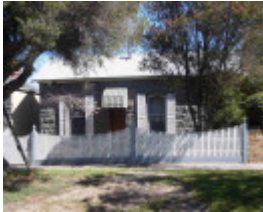
House at 17 Elizabeth Street NEWPORT, Hobsons Bay Heritage Study 2006
